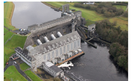
Hydro-Electric Power Station
